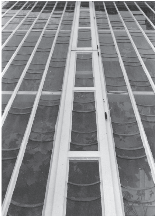
Paxtonian glasshouse detail.
